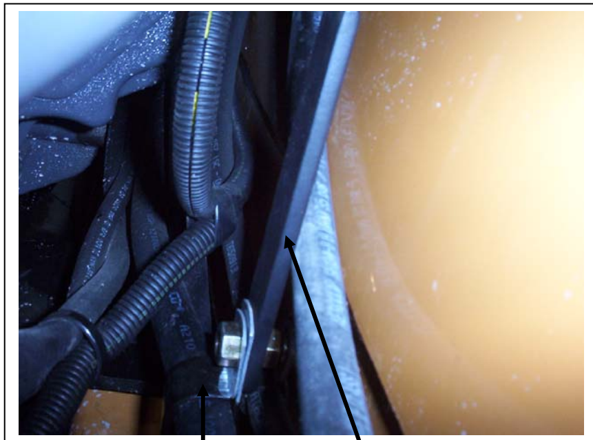
Heater hose bracket in the new location
