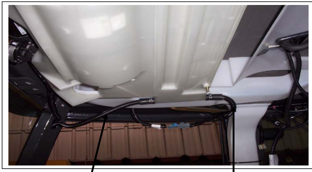
Front right drain tube
